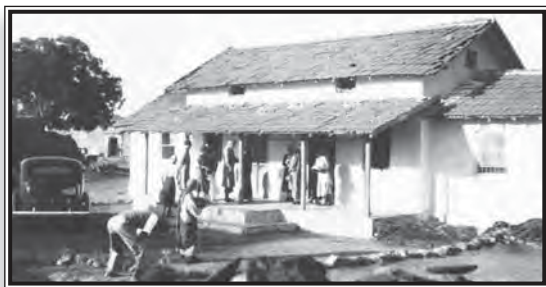
The "Family Quarters" at Arangaon village near Meherabad
