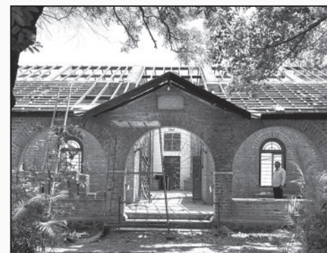
Front wing of MPC with roof open for repairs
