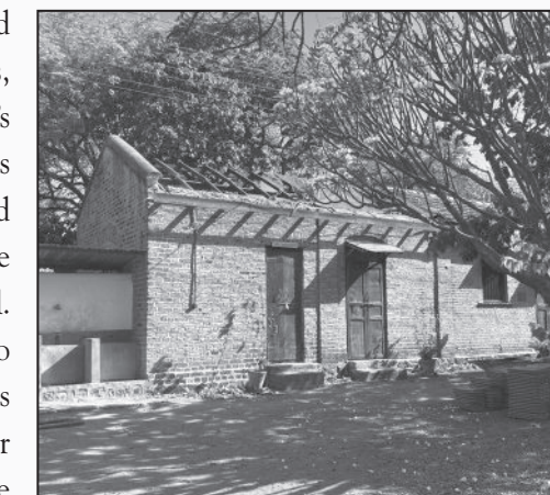
The kitchen building, roof under repair
