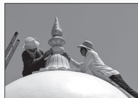
Working on the spire atop the dome
