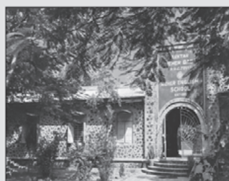
New roof panels seen to the left of the school entrance
