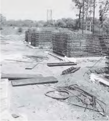
Work in process on the pedestrian underpass. Ten concrete sections are fabricated on site first. When they are ready, the railway line will be closed, and in a few hours workers will excavate below the track and insert the concrete
