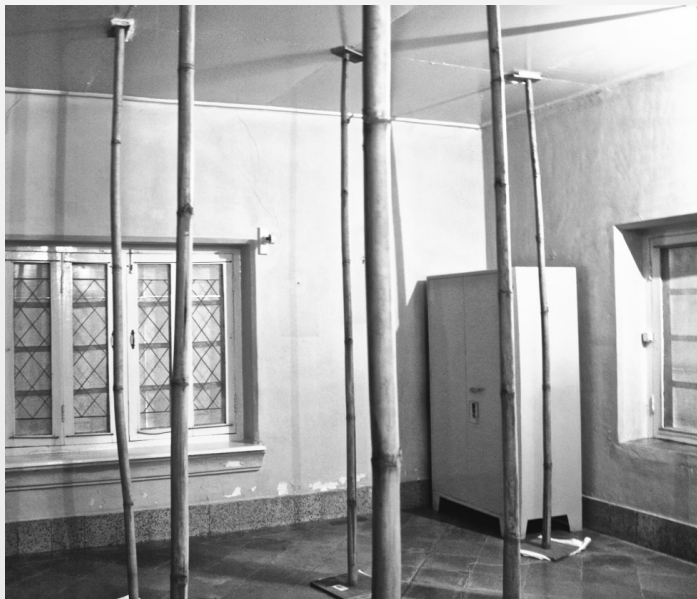
Baba's room fortified during construction.
